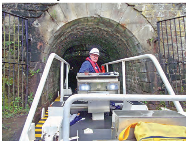
The rear tug pushing the specially built boat out of the Marsden end of the tunnel. Photo Adrian Armishaw
